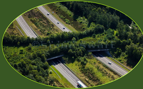
Ecoduct (wildlife bridge) on highway A1 through nature area the Veluwe, The Netherlands
